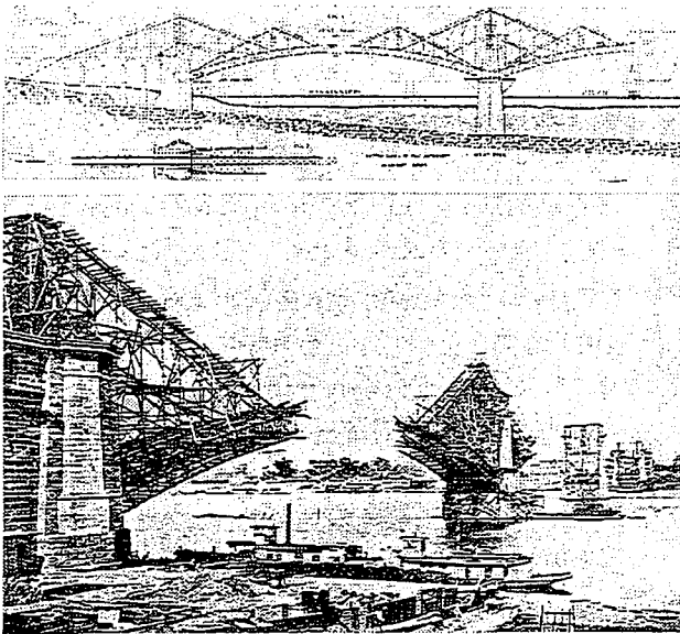
Photo.1 Construction of Eads Bridge (Completed in 1874) (Source : "Civil Engineering(Special Issue)" ASCE,1975 - 77,p.45)
